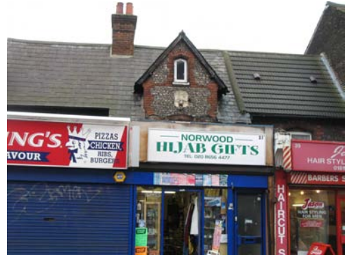
Picture 4.15 Distinctive flint - faced building
