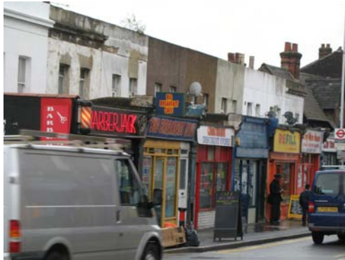
Picture 4.14 First floor is set back substantially from ground floor
