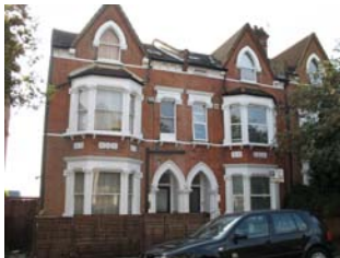
Picture 4.18 Locally Listed Building on Chalfont Road
