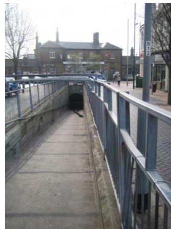
Picture 4.12 Norwood Junction subway and station, 2007
