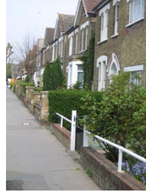
Picture 4.25 Residential Road built using London Stock. Very Well Preserved
